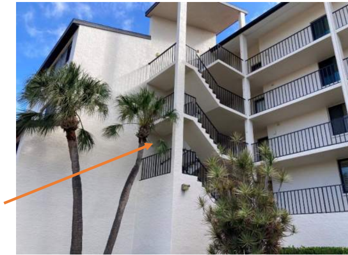
Figure 10: Typical Stairwall at Buildings 1 – 5
