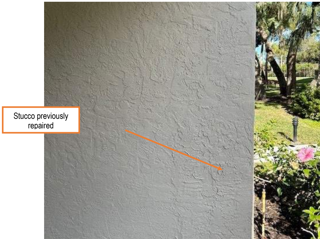
Figure 5: Monitor for delamination
