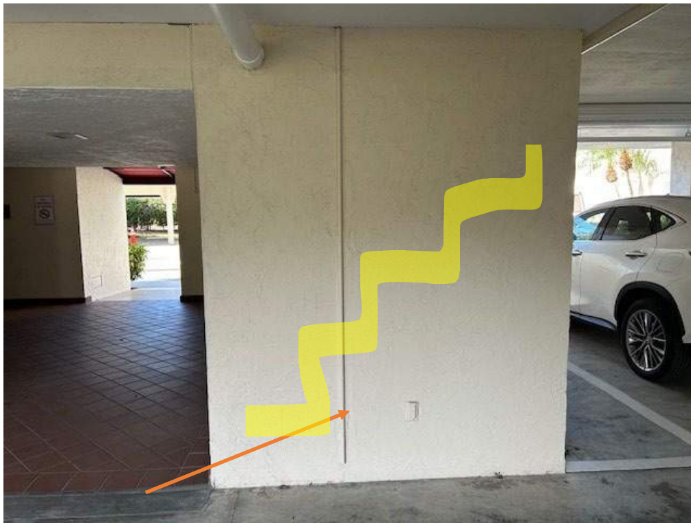
Figure 7: Stairstepping of CMU block in garage Typical
