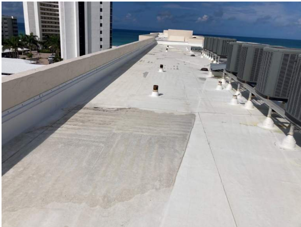
Figure 2: Roof at Gulf Buildings
