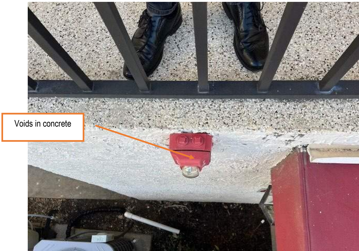
Figure 3: Opening at Strobes typical – apply sealant and fill void
