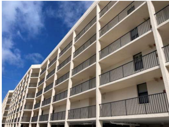
Figure 3: Columns at Gulf Building
